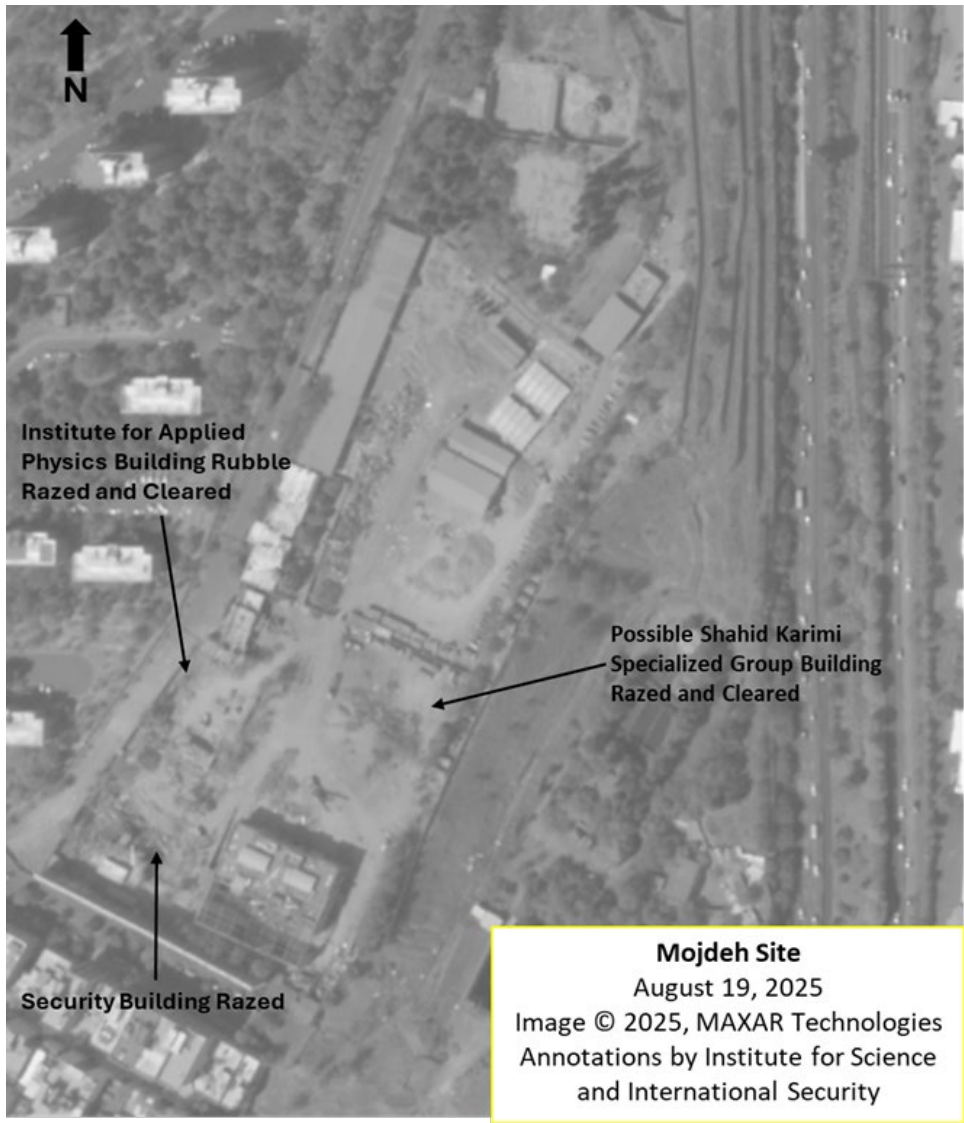
Figure 4. An August 19, 2025, MAXAR Technologies image of the Mojdeh site. Several buildings have been razed and cleared.
